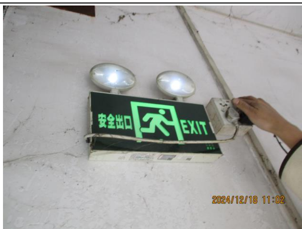
Emergency light test
