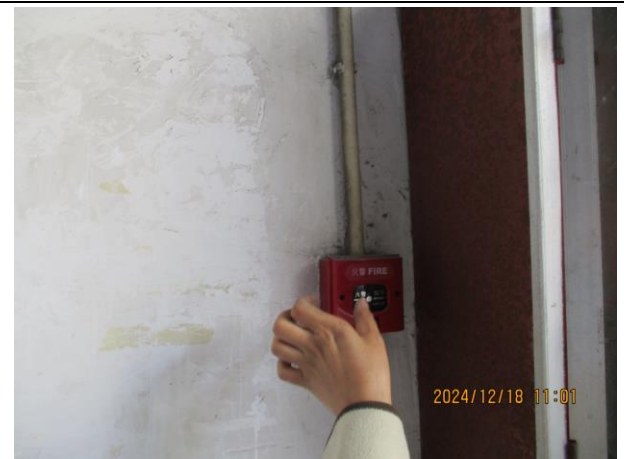
Fire alarm test
